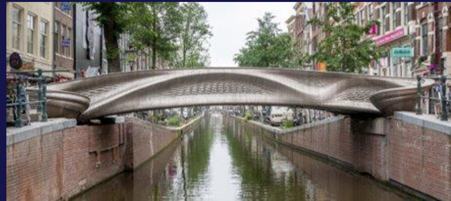
12-metre, 4.5-ton 3D-printed pedestrian bridge in Amsterdam
